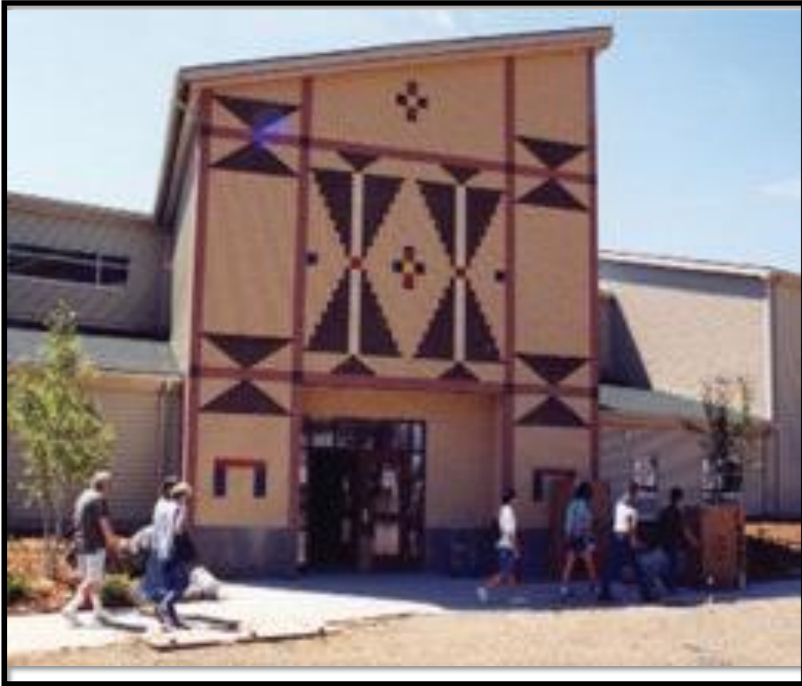
Driftwood Lodges Classroom Building at Little Big Horn College
